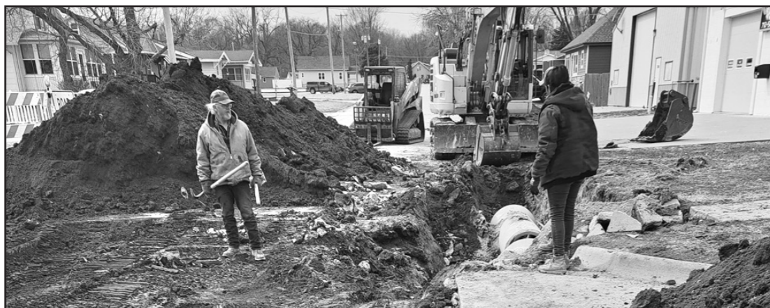
The resurfacing project includes sewer line work along Tyson Street.
